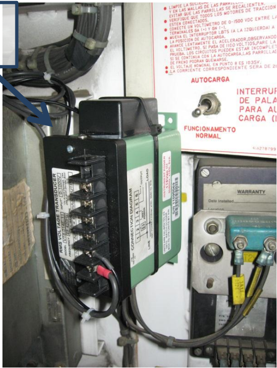
Figure 4 – Close Up of Voltage Transducer in Locomotive Electrical Cabinet
