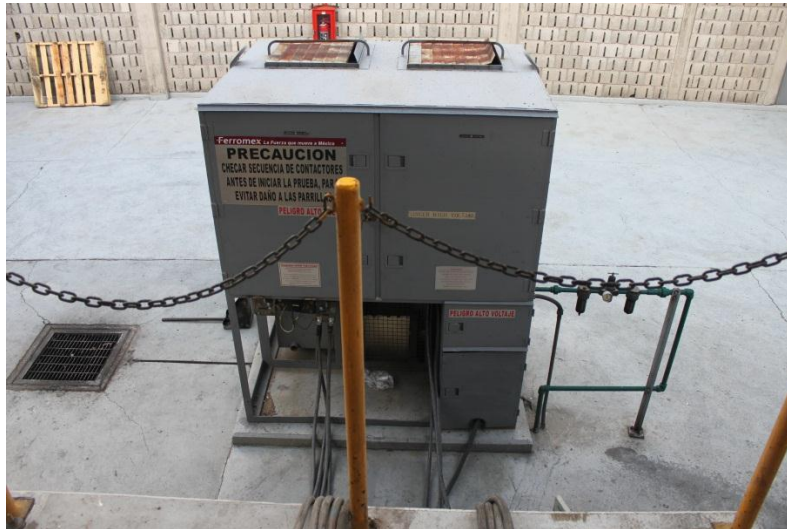
Figure 7 – Load Box used to Dissipate Power from Test Locomotive
